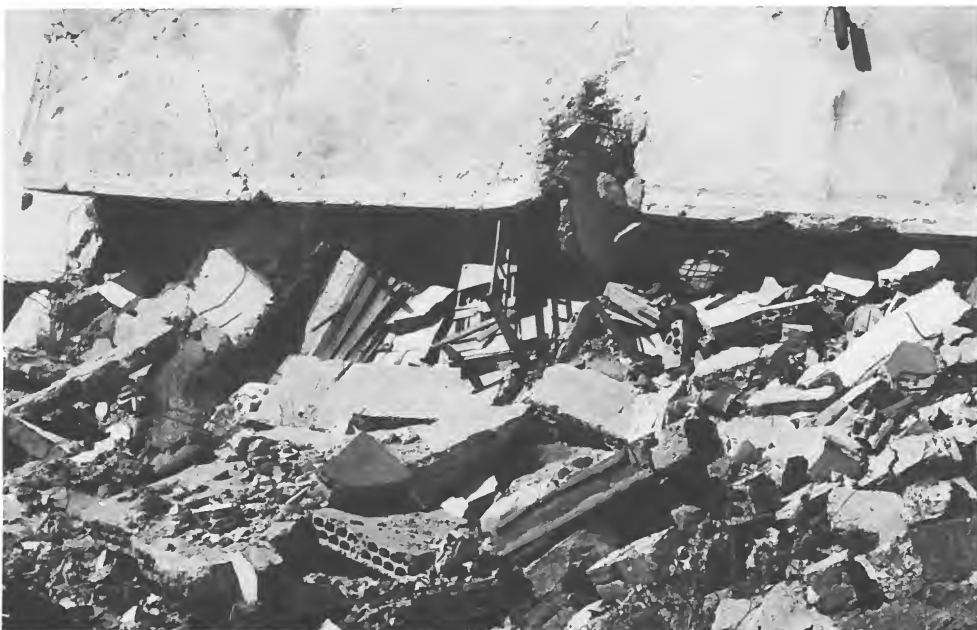
Ruins all around in preparation for building up more settlements. Israel's settlement policy aims at forcing the Palestinians to leave their land.
