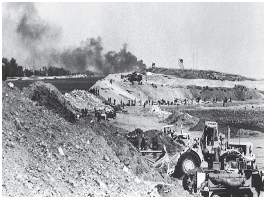
Mazmad Yard on the eastern bank of the Suez Canal, October 16. Courtesy of Shlomo Arad.
