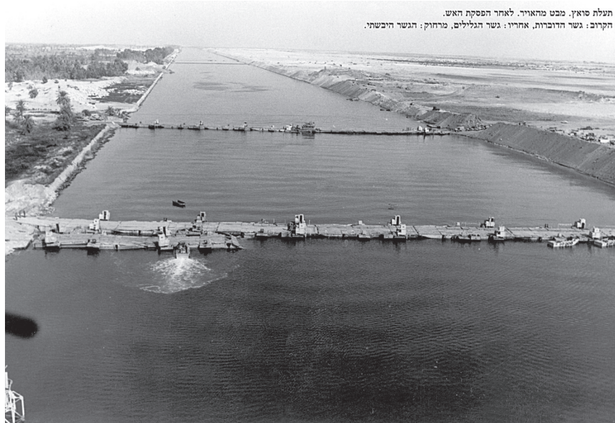
Diagonal aerial photo of the bridges on the Suez Canal ( looking south to north ), late December 1973. The raft bridge is shown in the foreground, followed by the roller bridge, and in the distance, the land crossing.
