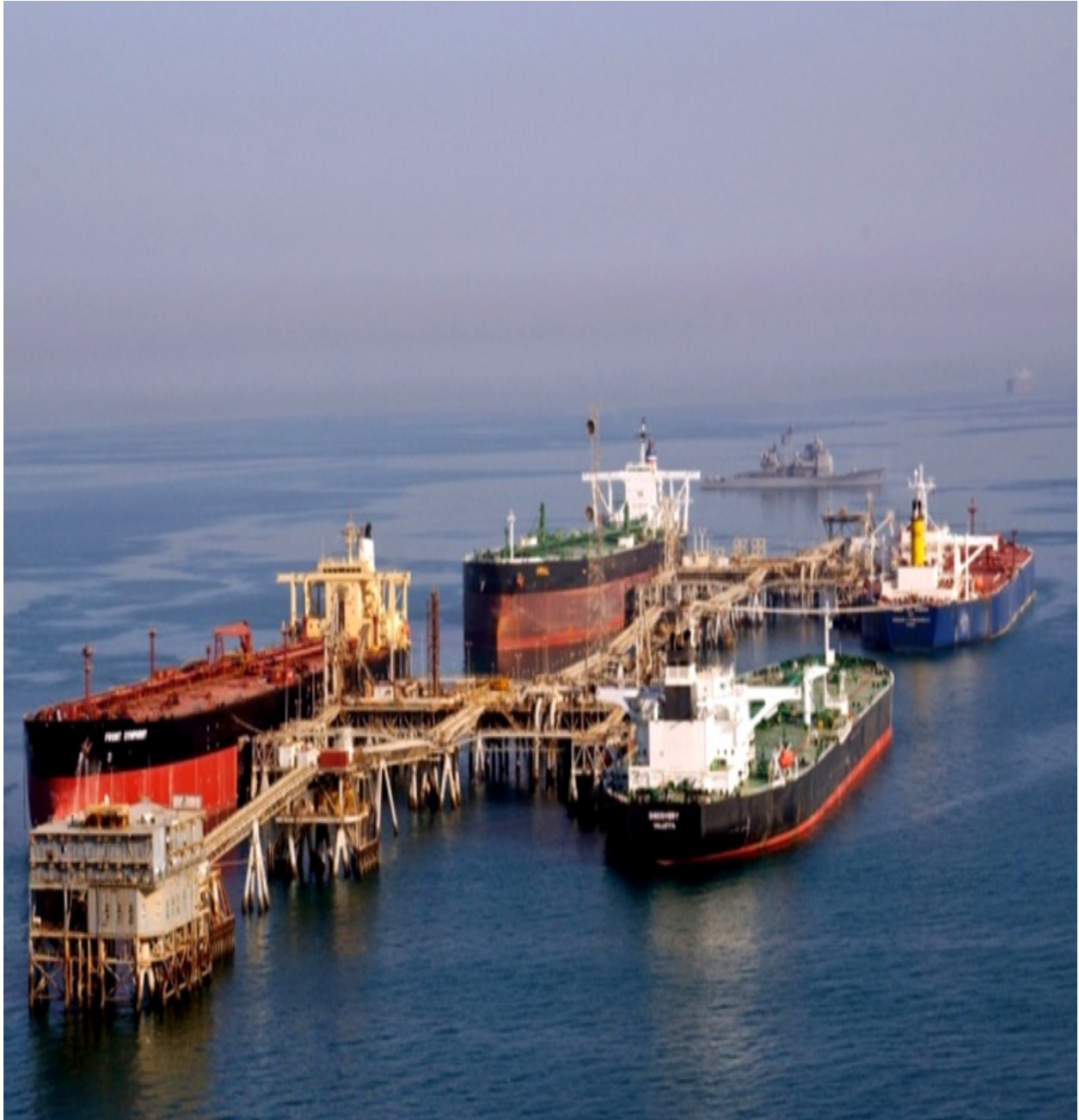
The Al Basra oil terminal loading four very large crude carriers; each ship carries 2 million barrels. The gray ship in the background is a US Navy cruiser providing security. Photo in public domain.
