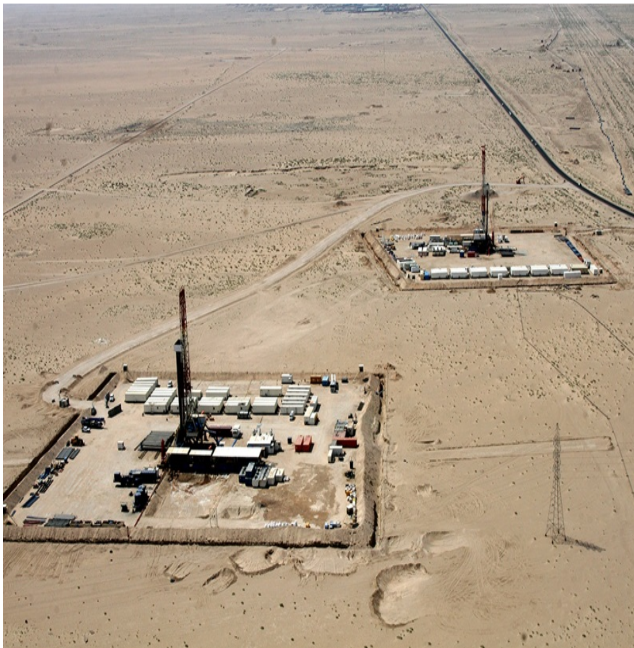
Two drilling pads with active rigs creating new oil wells in the Rumaila oil field, September 2011. Photo by author.
