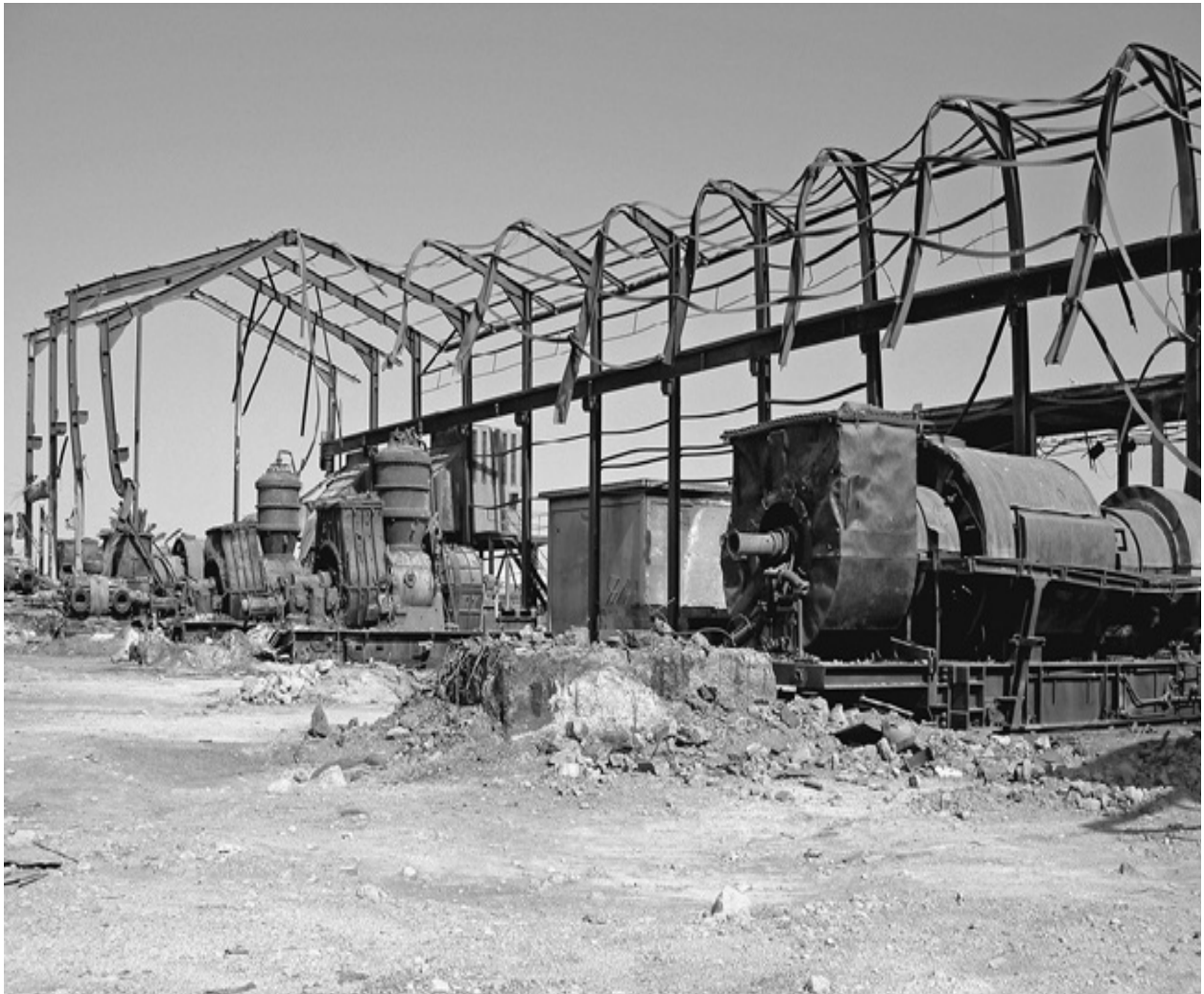
Gas turbine pumps and housing at the K-3 pump station destroyed in April 2003. Photo taken by Colonel Paul Dietrich USAR during a visit in 2006. Photo by Dietrich.
