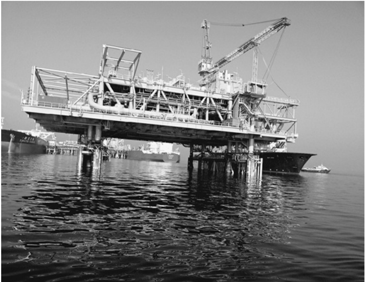
The central metering and manifold platform installed at the south end of the Al Basra oil terminal. Photo by Foster Wheeler.
