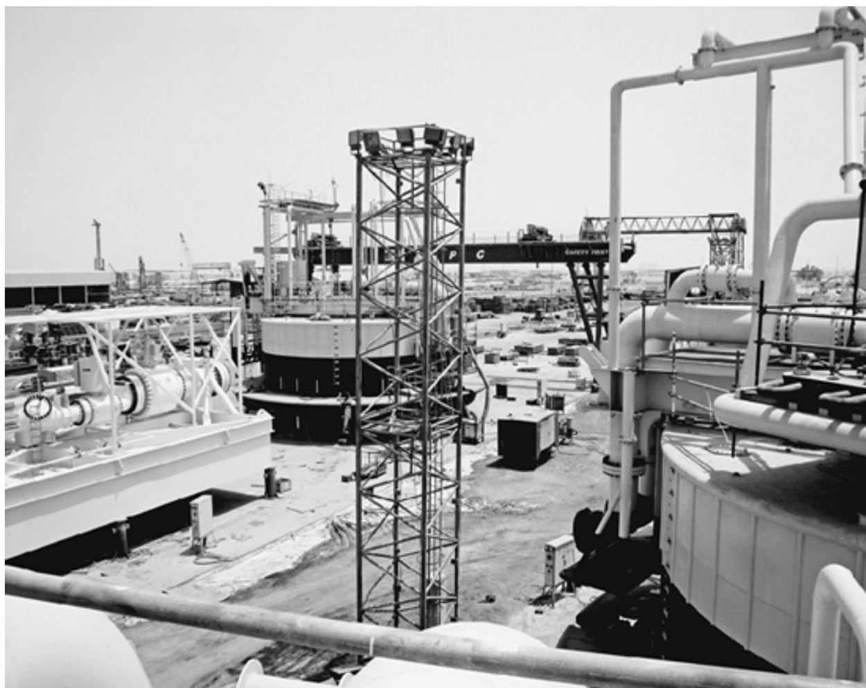
Single-point moorings (SPMs) in fabrication yard during August 2011. The light gray equipment on the left is a pipeline end manifold (PLEM) that is installed on the seabed under the floating SPM. Photo by author.
