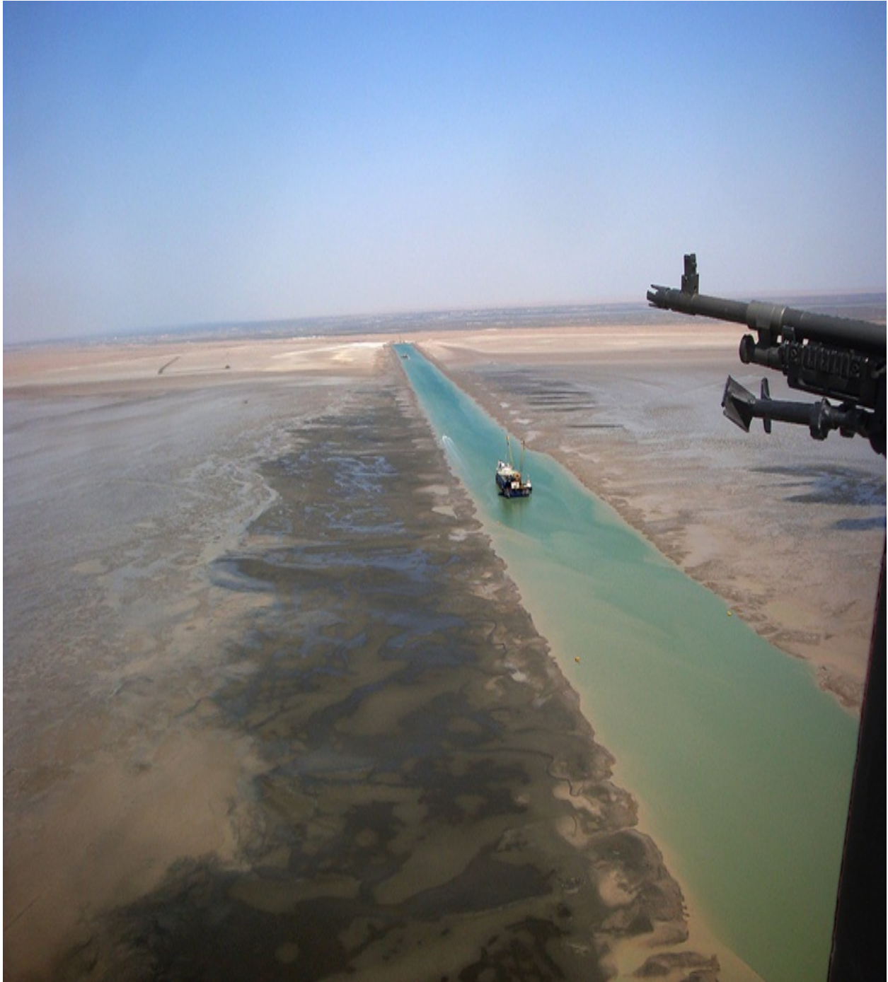
A pipe-laying barge is installing pipe from shore in a canal that had been dredged the month before our flyover in September 2011. The pipe is part of the export project that became operational in March 2012. Photo by author.
